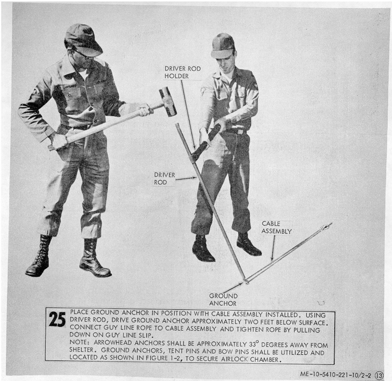
Figure 2-2(13). Erection of expandable shelter, (sheet 13 of 18).
