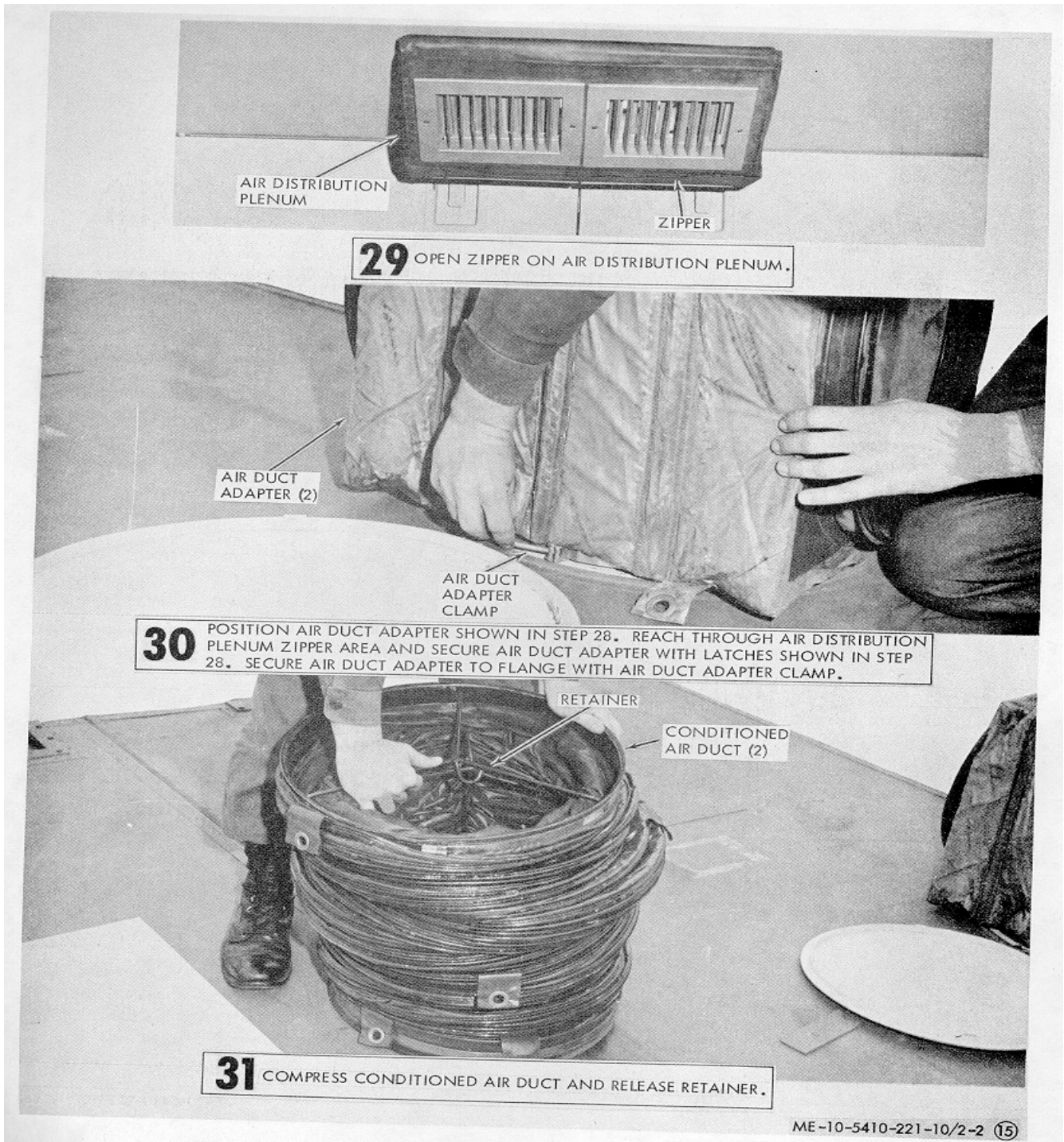
Figure 2-2(15). Erection of expandable shelter, (sheet 15 of 18).
