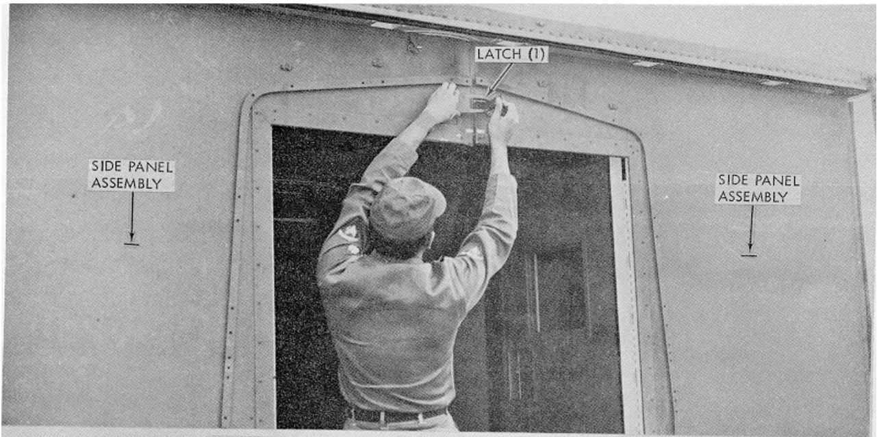
11 SECURE SIDE PANEL ASSEMBLIES TOGETHER WITH LATCH.
